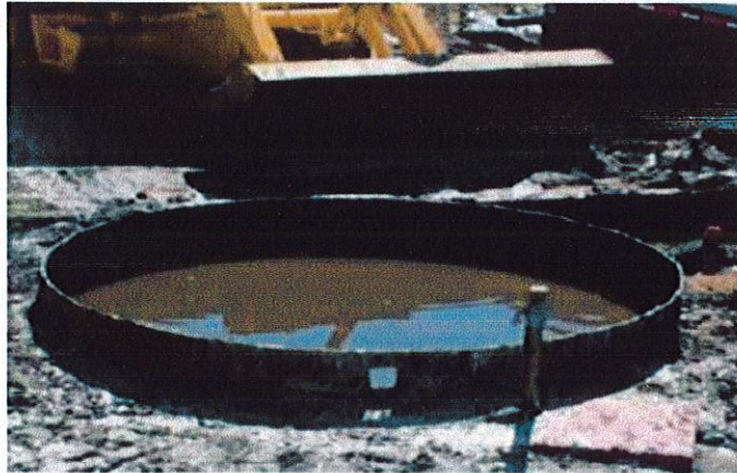
Figure 2. 4: Temporary Surface Casing Providing Containment for Slurry
